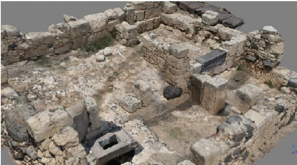
Fig. 4: 3D relief of the building n. 56 from South-East (from Fariselli et alii 2017a; relief and processing M. Marano).
