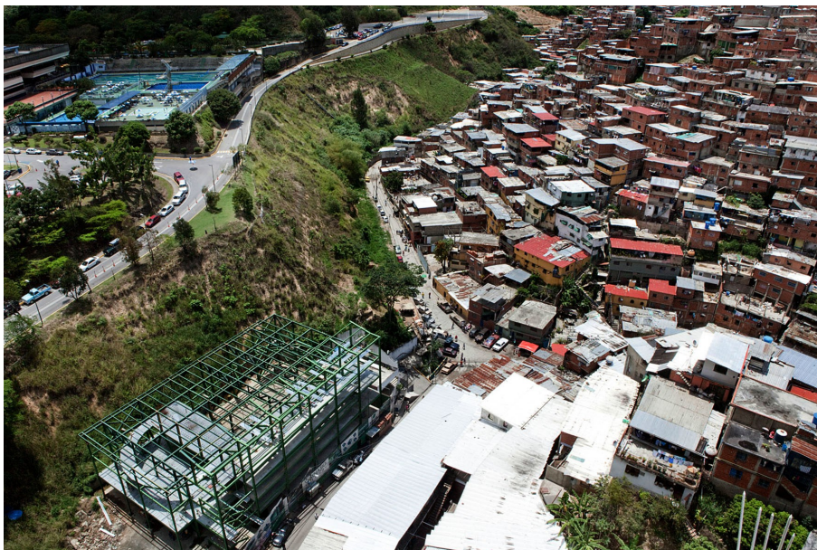
Image 3 - UT-T. Vertical Gym.Construction
